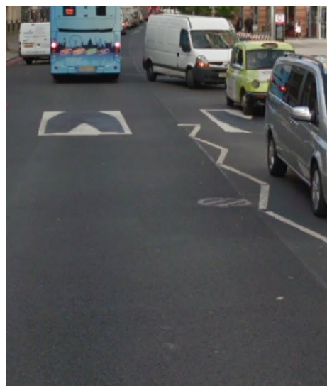
Flat “speed cushion” road marking in Southwark Street
